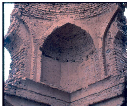
Figure 3: Hangu (Thal): Tor Gumbat, Showing Corner Squinch in Phase of Transition
